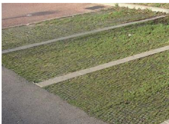
PLACES DE PARKING ENHERBEES NON ETANCHES (SOURCE GRAND LYON)
